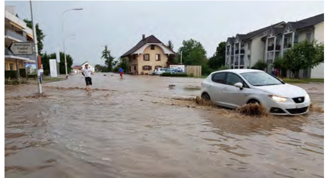
Abb. 3: Unwetter 2017 in Zofingen
